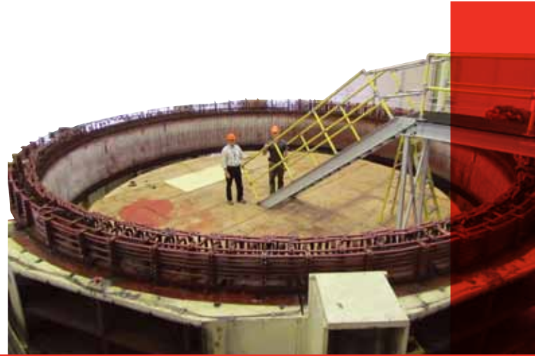
▲ Mountain Chute generator refurbishment to restore station's operating capacity in Renfrew.
